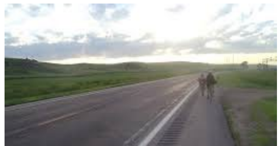
Figure 3-4: Paved shoulder with rumble strip. Source: Small Town and Rural Multimodal Networks , U.S. DOT FHWA.
