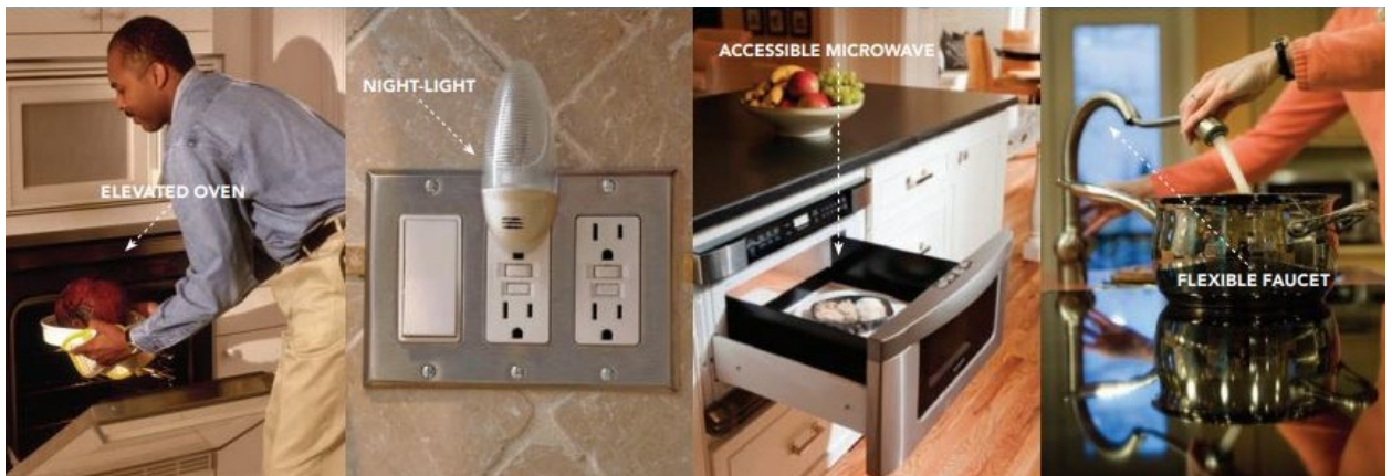
Figure 5-15: Examples of home features that increase accessibility and help people to age in place. Source: AARP HomeFit Guide.
