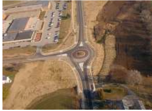
Lineville/Rockwell roundabout in Howard
